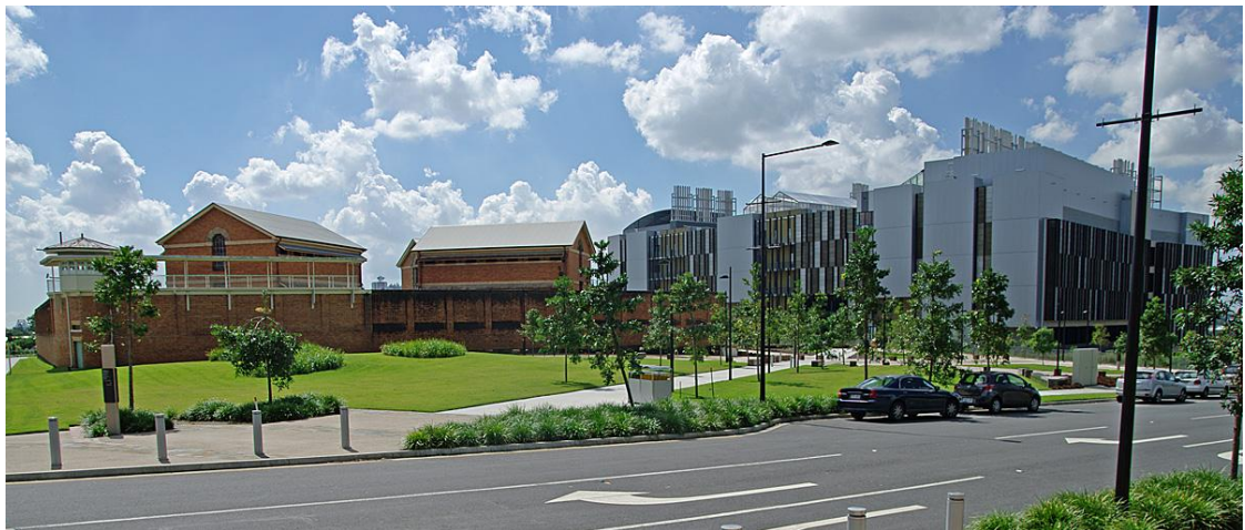
View of the old façade of Boggo Rd Gaol on the left with the new Ecosciences Precinct behind and to the right.
